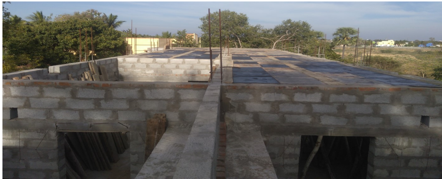
NEW BUILDING FOR THE SCHOOL FOR THE BLIND Begun in October '16. Below the support being laid (February 24) for the concrete roof on the second floor.
